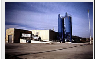
Since December 1989 N-Viro International Corporation has operated the City of Toledo's N-Viro Process facility that treats approximately 150 wet tons per day, or approximately 40,000 tons annually, of anaerobically digested sludge.
